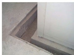
Excavation sample Dettaglio scavo
